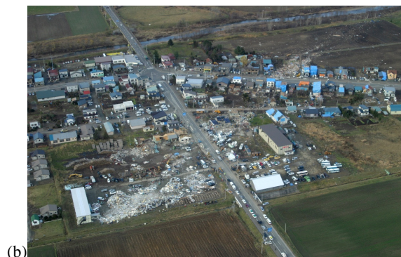
Photo 1 Damaged area of Wakasa, Saroma-cho. (Shin Engineering Consulting Co. Ltd.)
